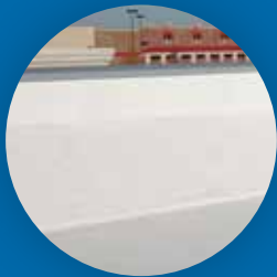
Custom-Fabricated Parapets and Wall Flashings
