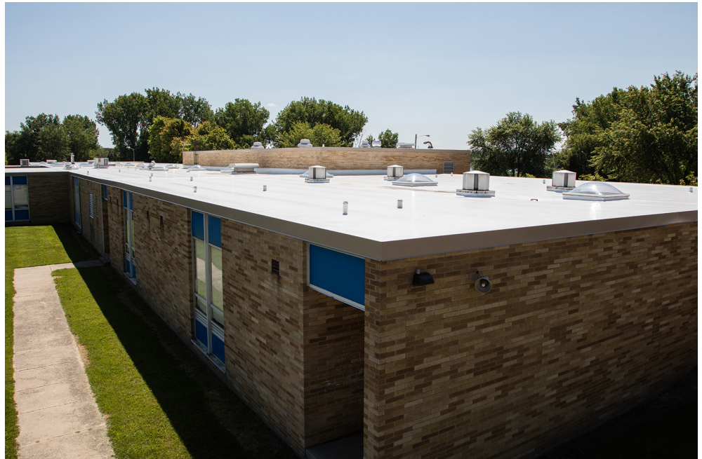
Studies show that cool roofing systems provide energy savings and other benefits when installed in cold climates. This cool roof was installed on West Shore Elementary School in Fenton, Michigan.
