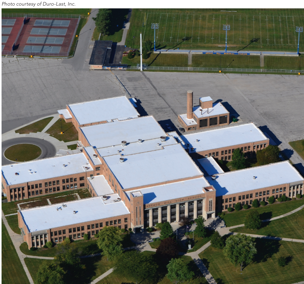
Cool roofs deflect solar energy away from a building and back to the atmosphere and beyond.
