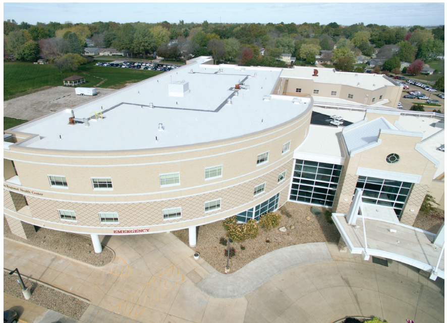
As medical facilities continue to expand to meet growing healthcare needs, so do their overhead costs. Enhanced insulation and reflective roofing investments provide valuable immediate and long-term savings opportunities that protect the bottom line and patient care. Photo courtesy of Duro-Last.
