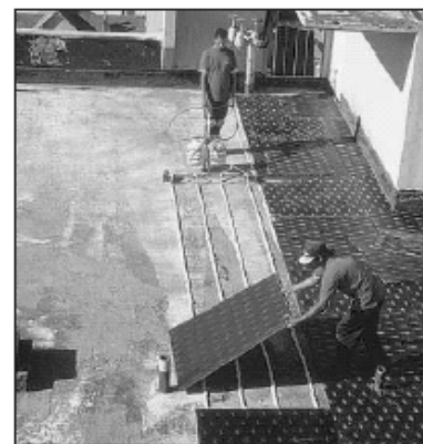
Figure 3: Installation using MBA
